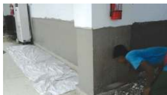
Town Hall, Kolkata: Application Work in Progress
